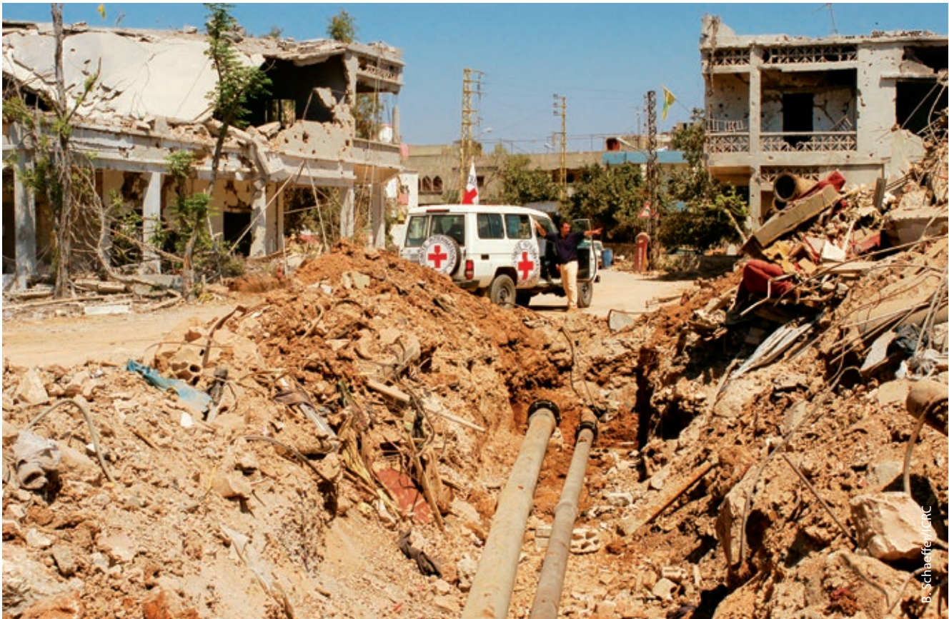
Photo 3. Direct and indirect impact starting to accumulate. It may be possible to repair these pipes but if water pressure remains insufficient, local residents are likely to install suction pumps – a “negative” coping mechanism that places the health of many more people at risk. (Southern Lebanon, 2006)
