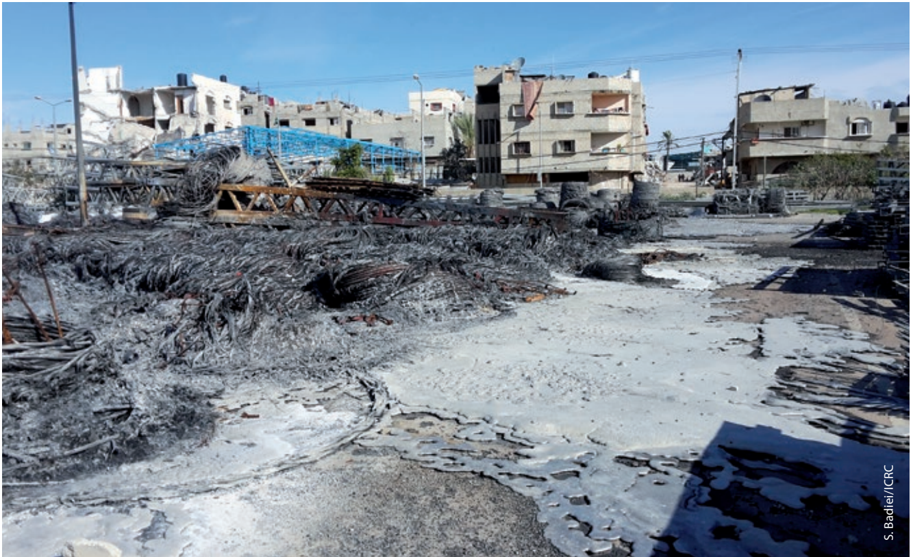
Photo 5. Melted wires and poles resulting from the destruction in 2014 of the warehouse of the electrical company of Gaza, which lost its capacity to react to breakdowns. Necessary repairs to the electricity grid had to be carried out by dismantling items such as transformers, wires and poles at less critical places and placing them in more critical places (e.g. hospitals). (Gaza, 2014)
